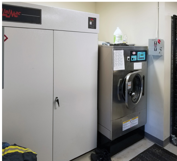
Failure to plan proper spaces in a firehouse's decon laundry area can lead to equipment being installed in a way so that it can't be repaired without the removal of both the disconnect and the machine.
