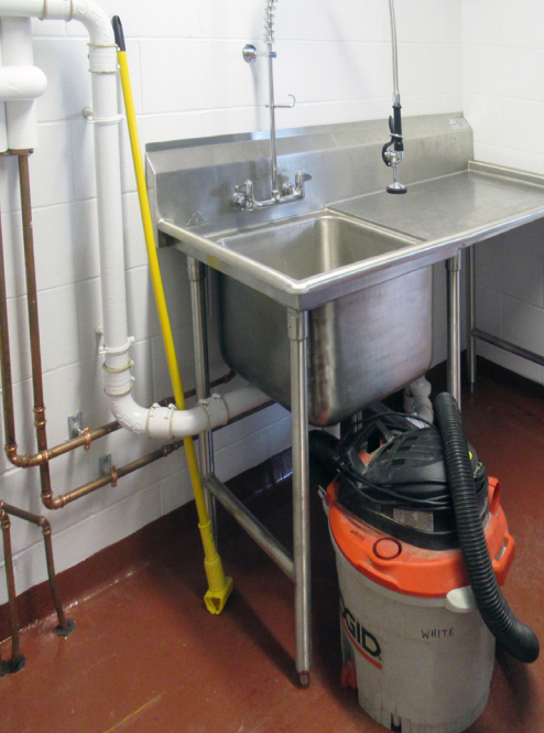
Failure to plan plumbing and bury it in the wall leaves a room impossible to keep clean.
