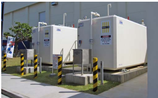
Bollards are a common hardening tool, as they prevent vehicles from ramming the facility. Photo by Les Edmonds/Komatsu Architecture
