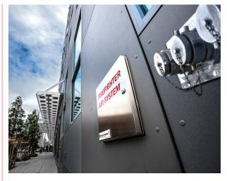
You need two things to fight a fire: water and air. Water standpipes have solved the problem of providing water inside complex structures. FARS solves the problem of air delivery.
