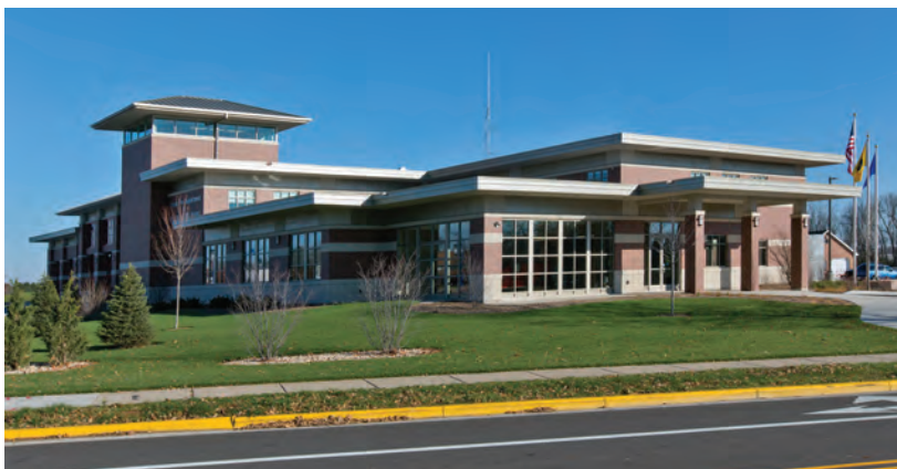
A station site must be located on, or adjacent to, a main travel artery that provides good access, egress and visibility for responding fire department emergency apparatus.
