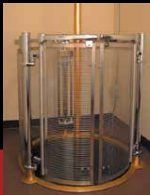
Model 23 for fire separation and protection of hole
