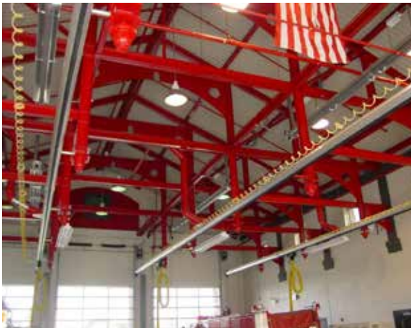
Charlotte, NC, Station 34 features a truck bay with decorative hydrant caps overhead. Photo by David Hartman
