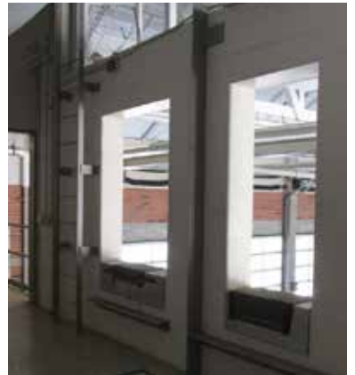
These windows are used for bailout and firefighter rescue training.
