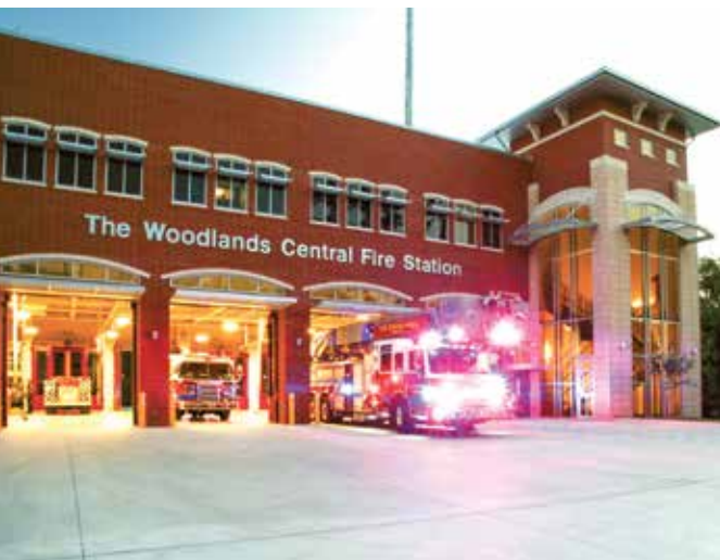
The Woodlands Township Fire Department's Central Fire Station is a two-company firehouse with fire apparatus, EMS units, fire administration, dispatching and an emergency operations center. Photo courtesy of The Woodlands Township FD
