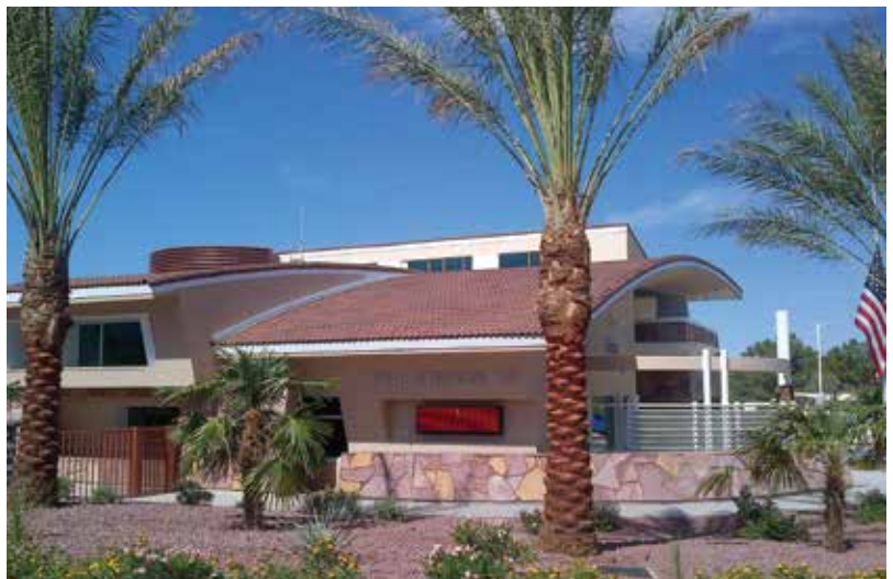
Las Vegas, NV, Fire & Rescue Station 107, which was constructed in the Sun City Summerlin senior citizen community, is Leadership & Energy Efficiency Design (LEED) Silver certified.
