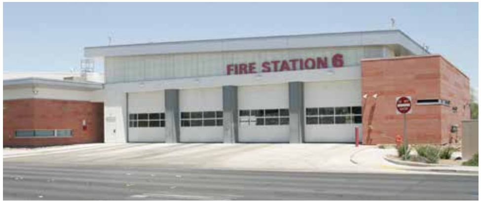
Las Vegas Fire & Rescue designs its fire stations with simple roof lines to keep initial costs down and make maintenance easier and more affordable. The department prefers metal roofs or single-ply membranes. Photo courtesy of LVFR
