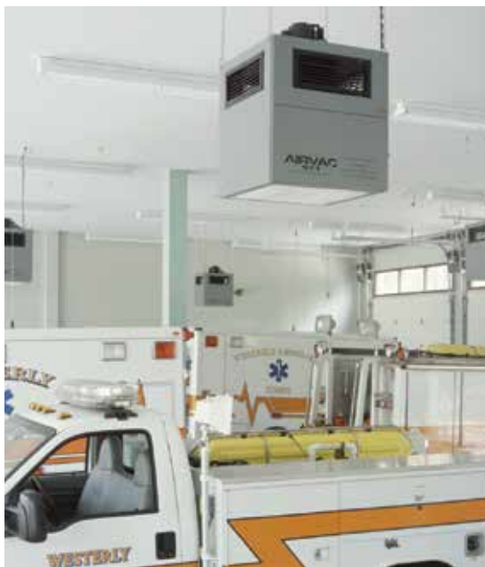
The AirVac system is completely automatic with no hoses to attach to apparatus.
