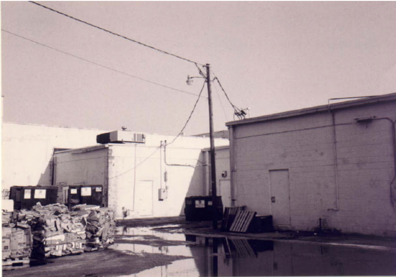
Utility pole connecting power to a meter at the rear of the Indian River Shopping Center. ( USFA file photo. )
