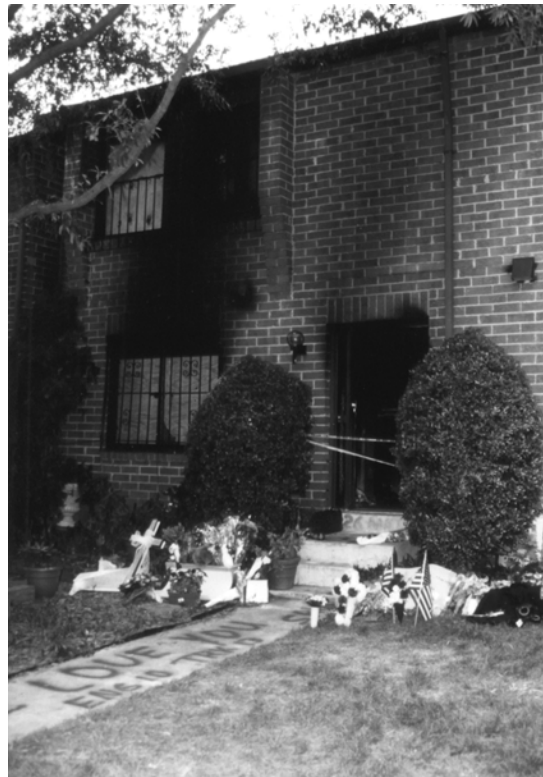
Photo 1 Front of 3146 Cherry Road, N.E.
