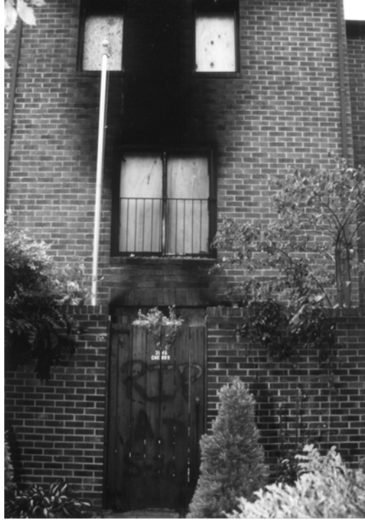
Photo 2 Rear of building as viewed from outside the patio fence.
